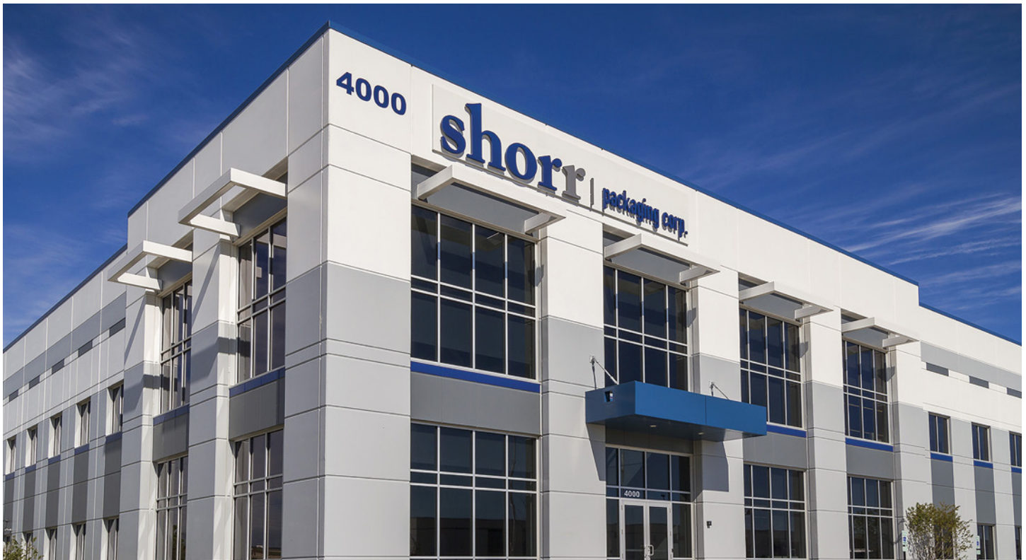
Shorr Packaging Corp's newly constructed corporate headquarters opened in Aurora, Illinois, earlier in 2016.
